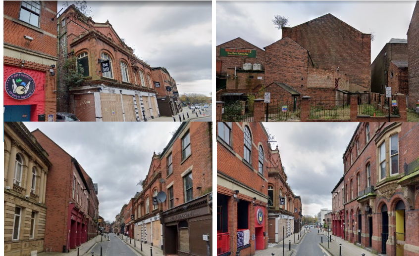
Figure 5-8: King Street Frontage (Top Left) Library Street rear (Top Right) King Street (Bottom) [Source: Google Maps]
