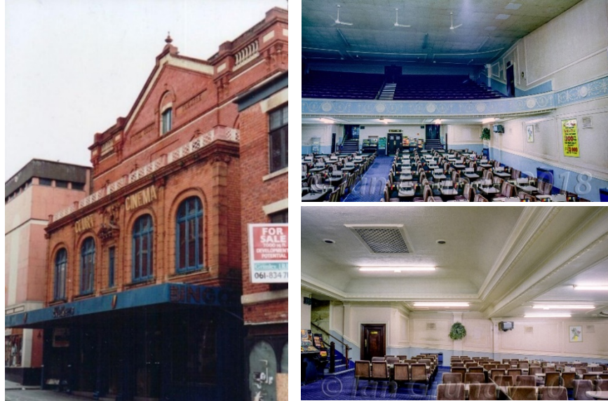
Figure 17-19: County Bingo Hall from King Street c.1990's (Left) Interior from stage (Top Right) Interior from Stalls (Bottom Right) [Source: Ron Hunt, Ian Grundy wiganworld.co.uk].
